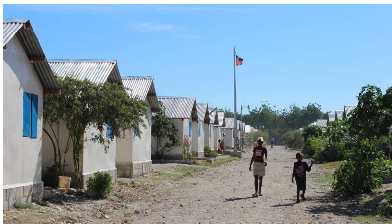
IOM Shelter units constructed in Santo 17 in Croix-des-Bouquets
