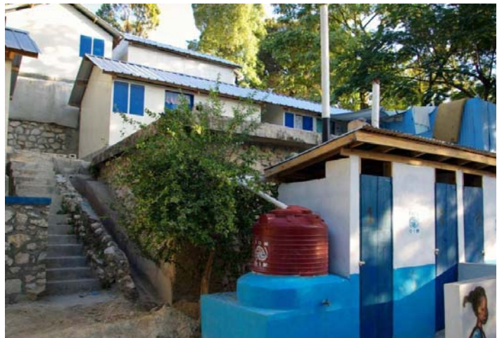
IOM Shelters constructed in Morne Lazare
